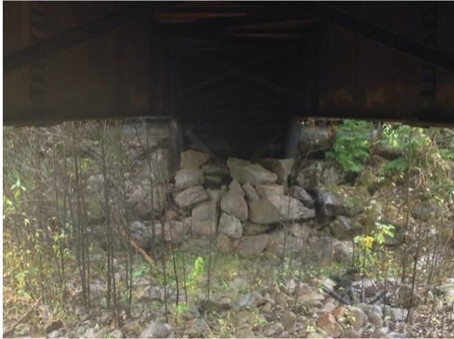
Left Bank Abutment when facing downstream
