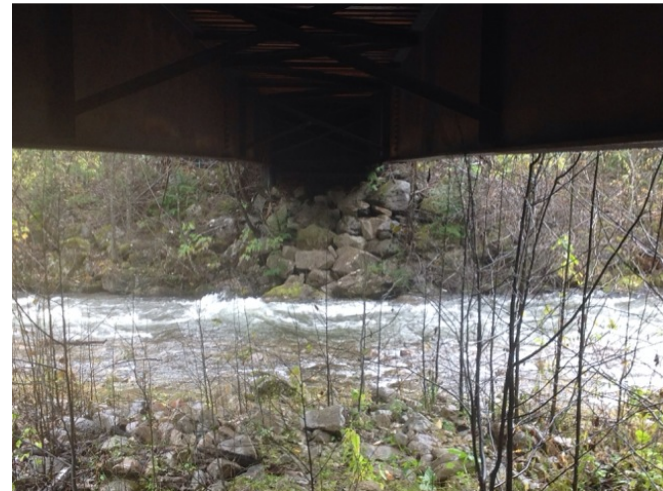
Right Bank Abutment when facing downstream
